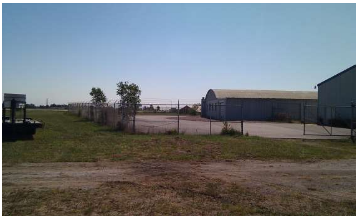
Parking area on landside of Bandag/Bridgestone hangar (E1 on terminal area plan).
