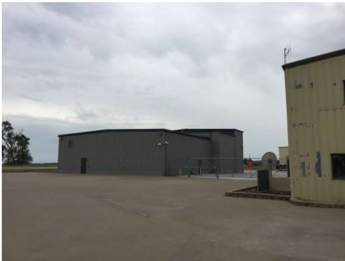
Parking area on landside of GPC hangar (E12 on terminal area plan).
