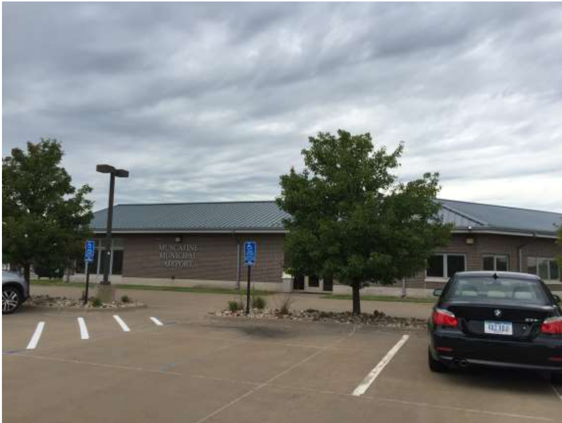
Looking north towards terminal building from terminal building parking area
