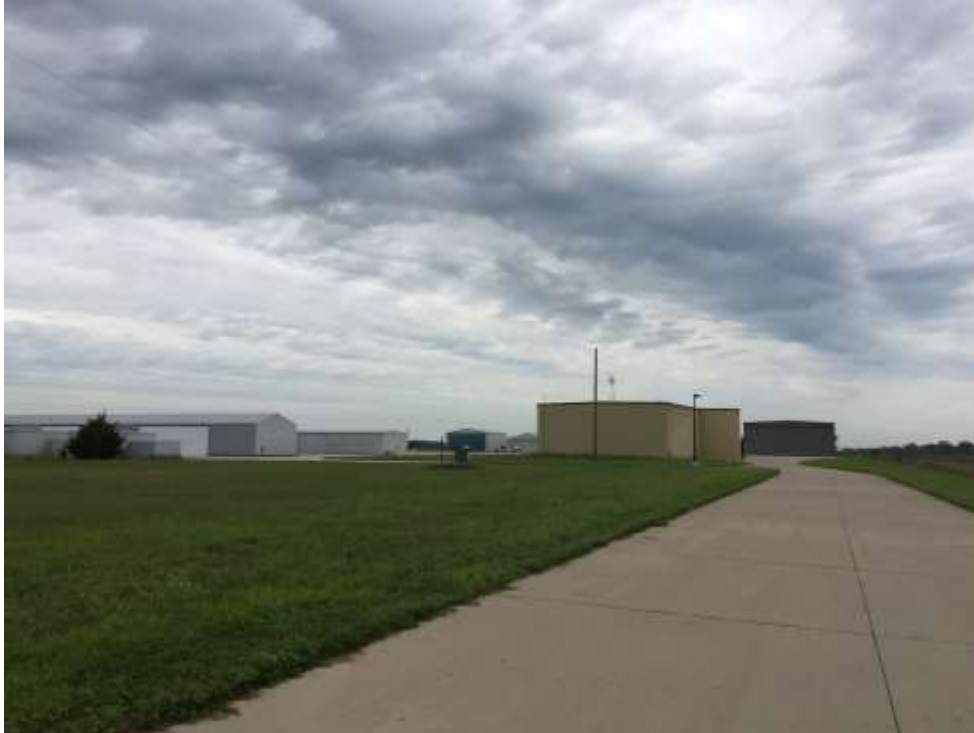
Looking east from the frontage road at the site of future conventional-style hangars
